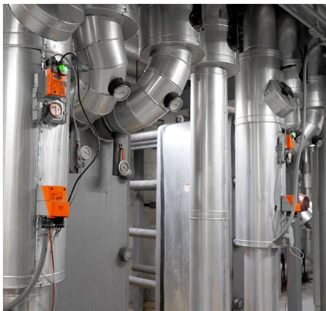
The Belimo Energy Valve is an IoT cloud connected pressure independent valve that monitors coil performance and energy consumption while maintaining Delta T. © Arboleda
