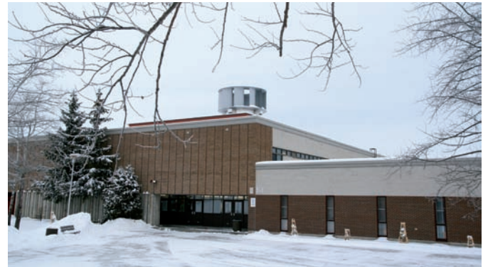
St-Roch-de-L'Achigan School with wind turbine.
