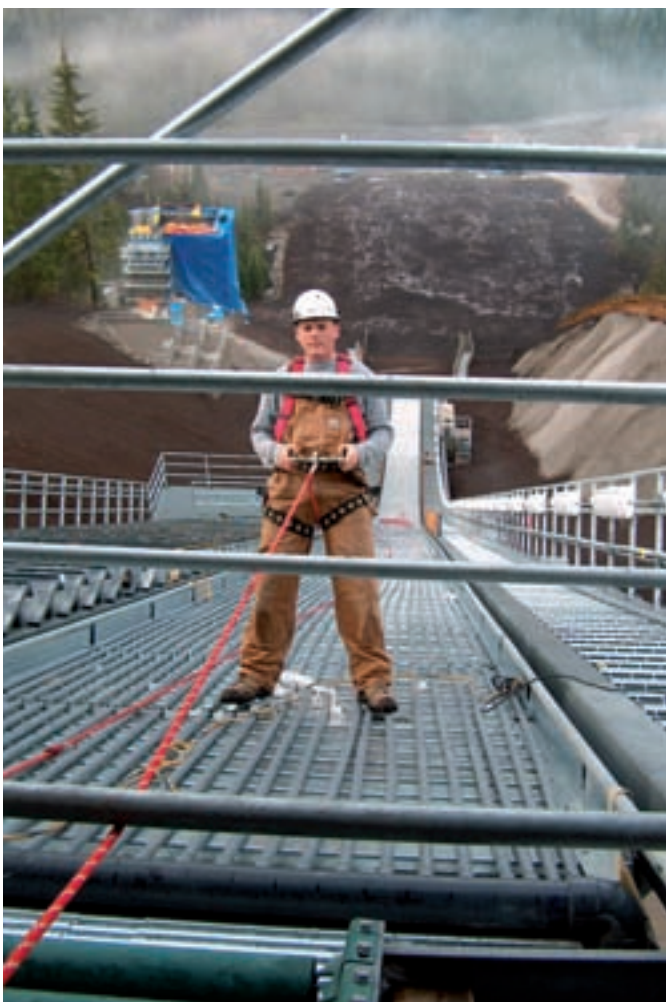
The mechanically cooled ski jump construction has a height of 125 meter.
