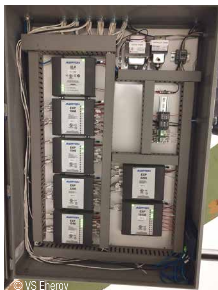
© VS Energy Alerton AAC - Advanced Application Controller with expansion modules for the central chilled water plant
