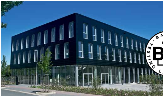
The DIAL building, Lüdenscheid: The architecture and overall technical concept were developed in-house. © DIAL
