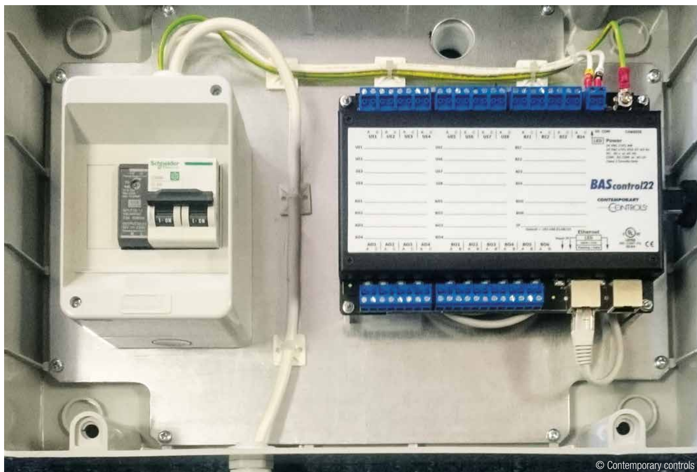
The BAScontrol22 provides the BACnet interface for people-movers at Manchester Airport.
